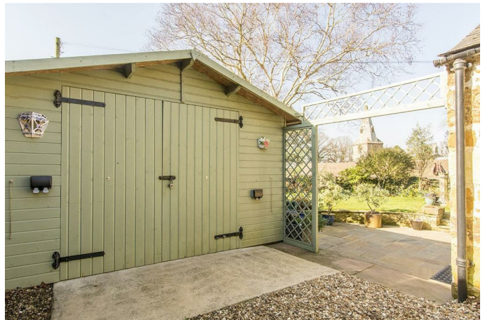
Timber double vehicle access doors. Power connected.
